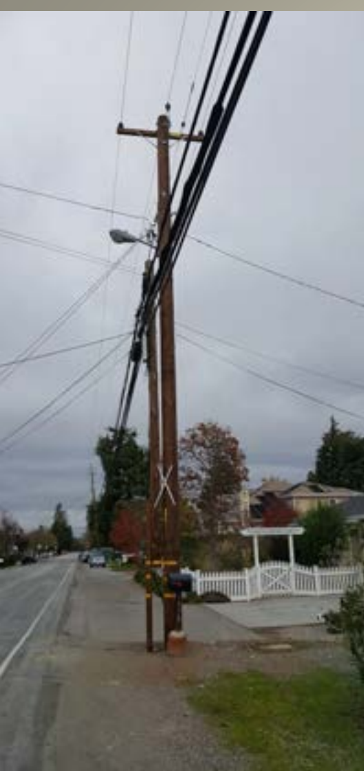
Photos showing "Buddy pole" created by PG&E while telecom equipment delayed transition and pole after equipment properly moved following utility Pole Tour led by Professor Sandoval in May 2018
